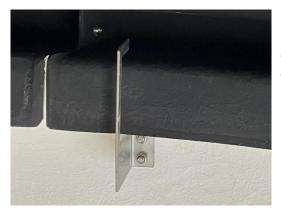
Make sure there is equal clearance top and bottom of the dome flange before marking and fixing the clamps and make sure that the dome top rotates freely without hitting any clamps and adjust if necessary.
